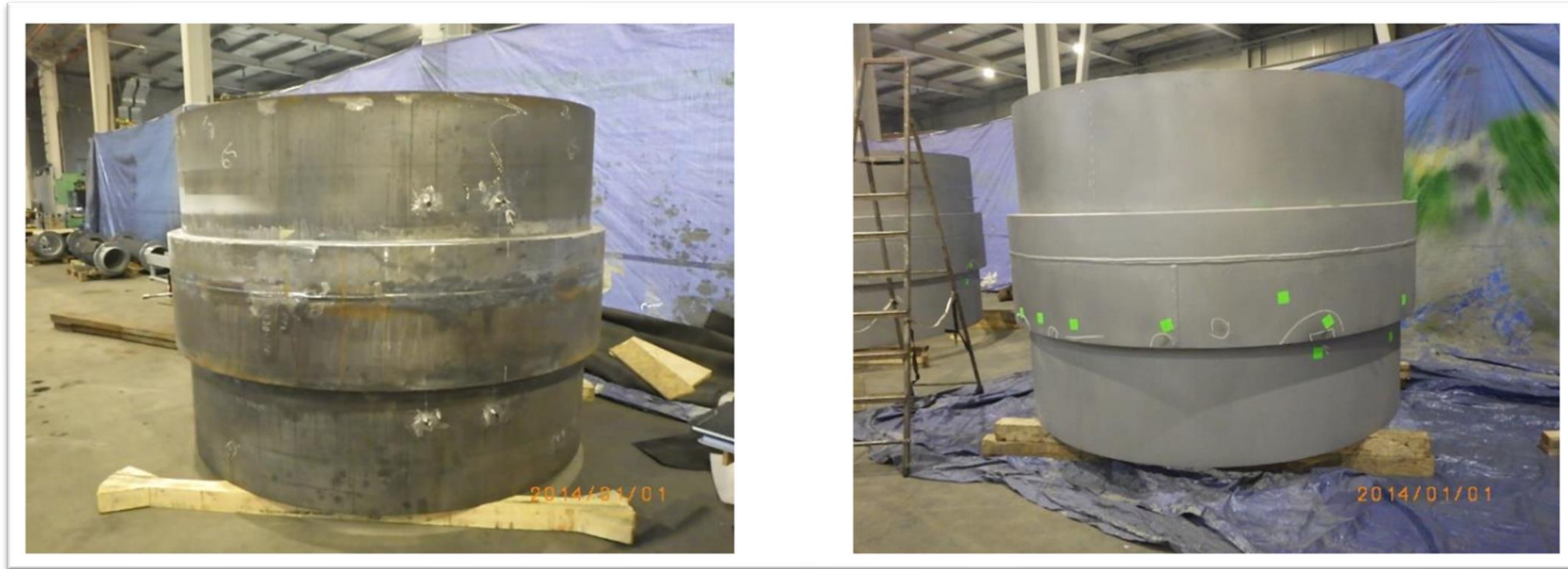
Surface blast (prep for coating)
