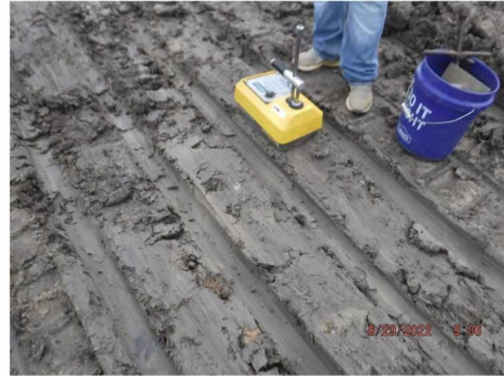
Pipe Embedment and Backfill Density Testing
