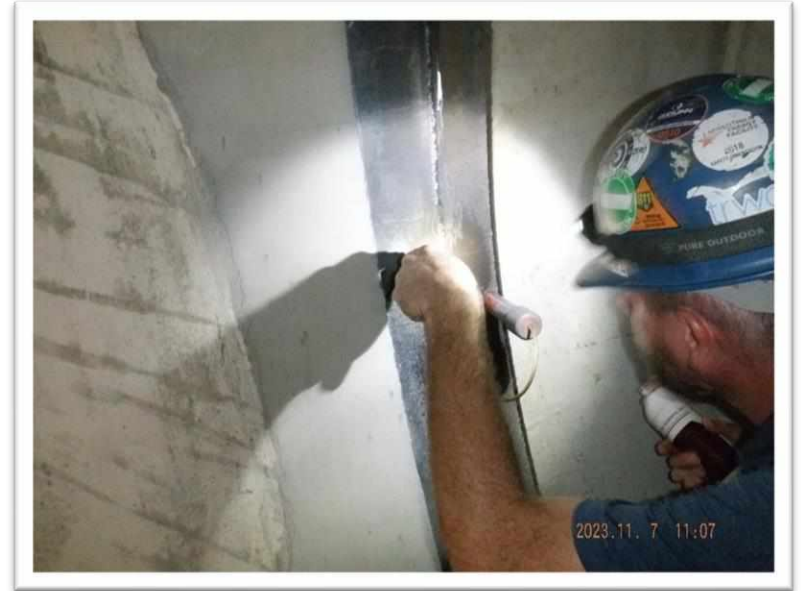
Magnetic Particle Testing Lap Joint Welds
