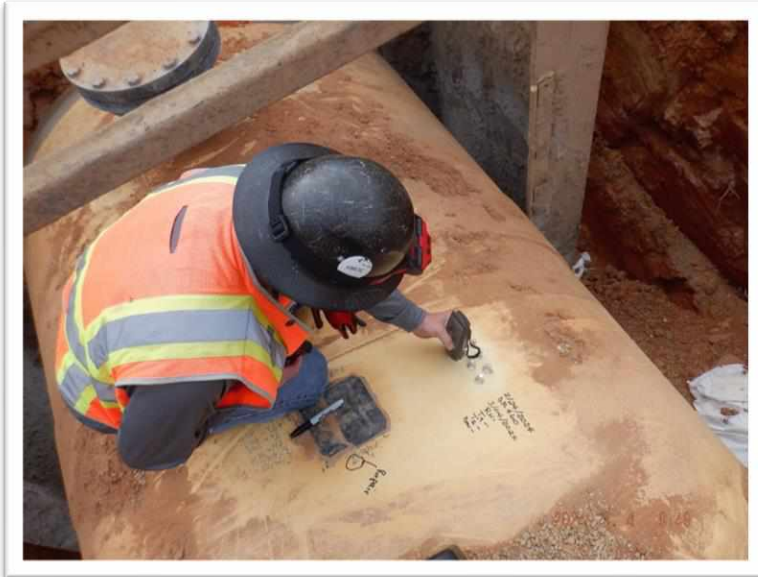
Pipe Coating Thickness and Adhesion Testing
