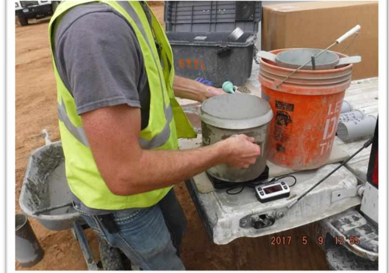
Unit Weight Test for Annular Space Grout
