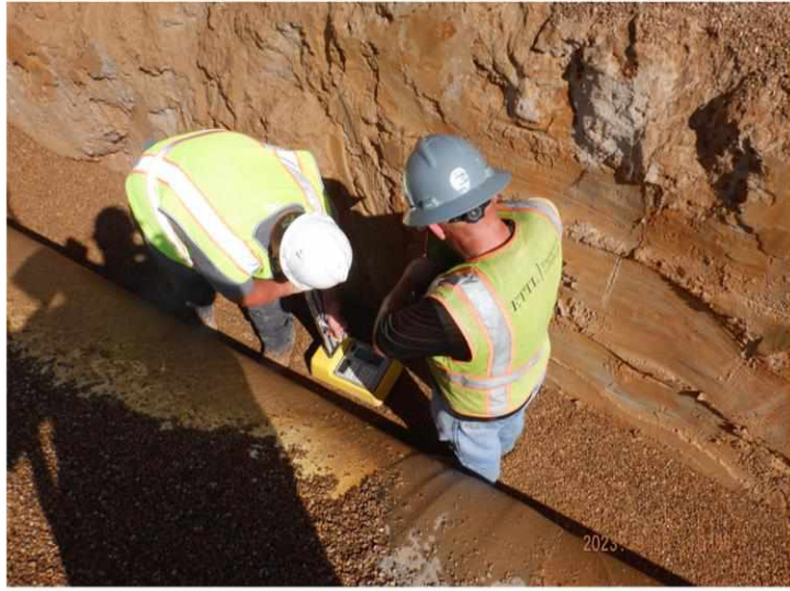
Pipe Embedment and Backfill Density Testing
