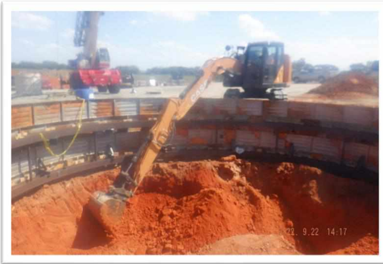
Production Inspecting/Monitoring Tunnel Shaft and Tunnel Excavations
