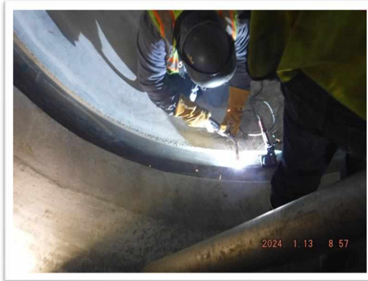
Welder Prove Out Oversight
