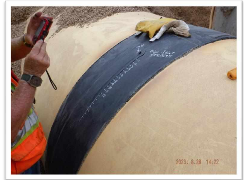
Heat Shrink Sleeve and Weld-After-Backfill Testing
