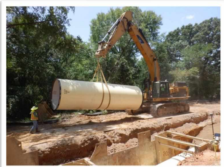
Production Inspecting/Monitoring Pipe Embedment and Backfill
