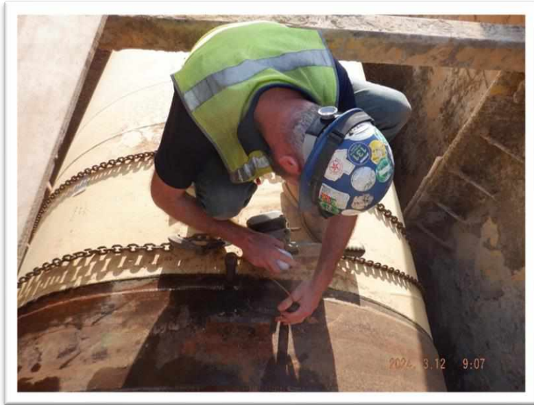
Air Testing Butt-Strap Joint Welds
