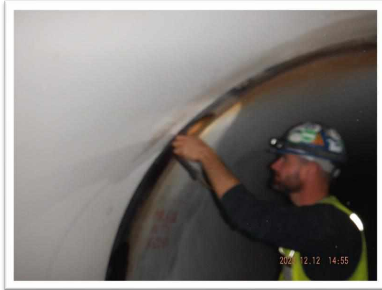
Visual Inspection Lap Joint Welds
