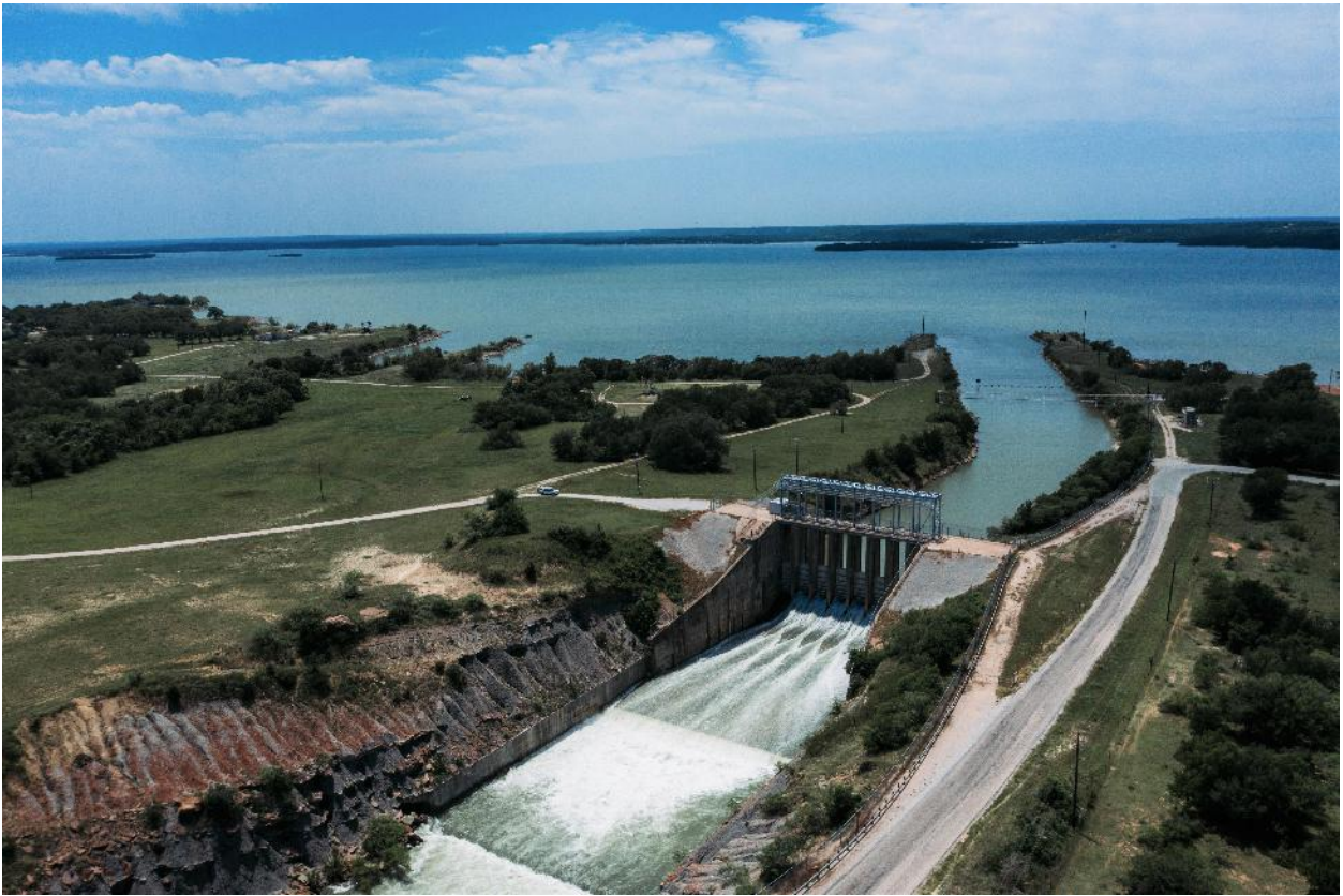
(Dam on Lake Bridgeport)
