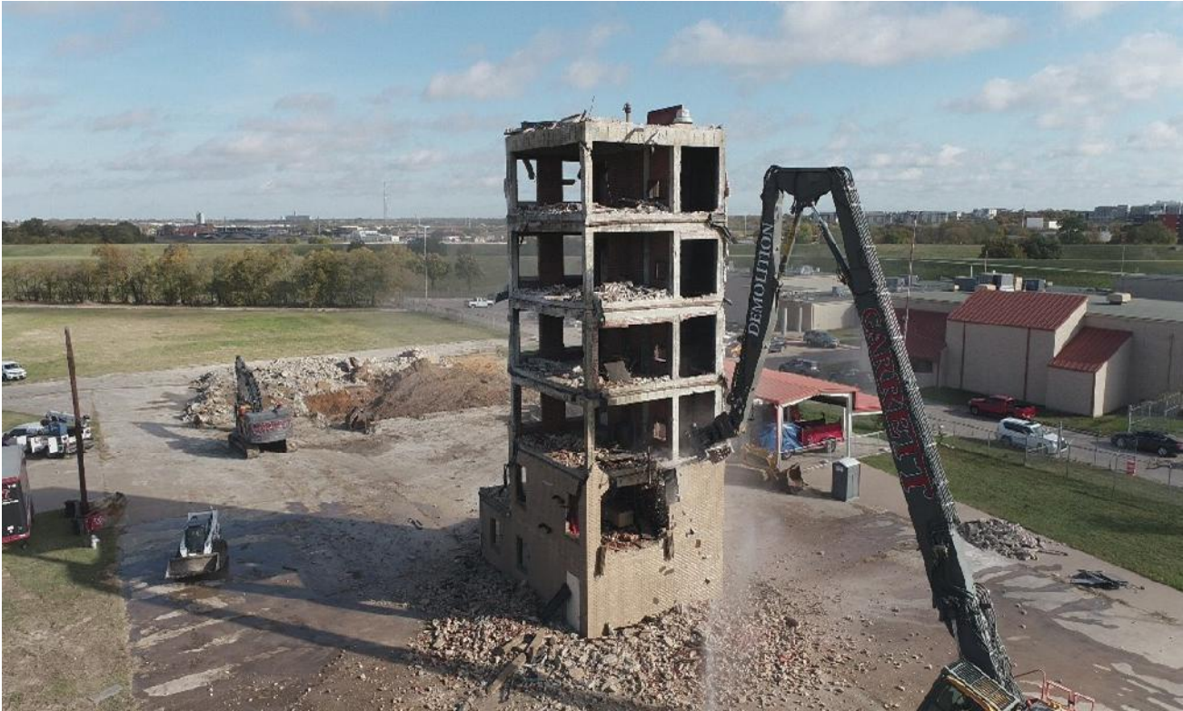
(Demolition of Police and Fire Towers)
