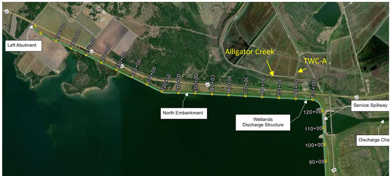
Figure 1: Overview of Richland Chambers – North Embankment
