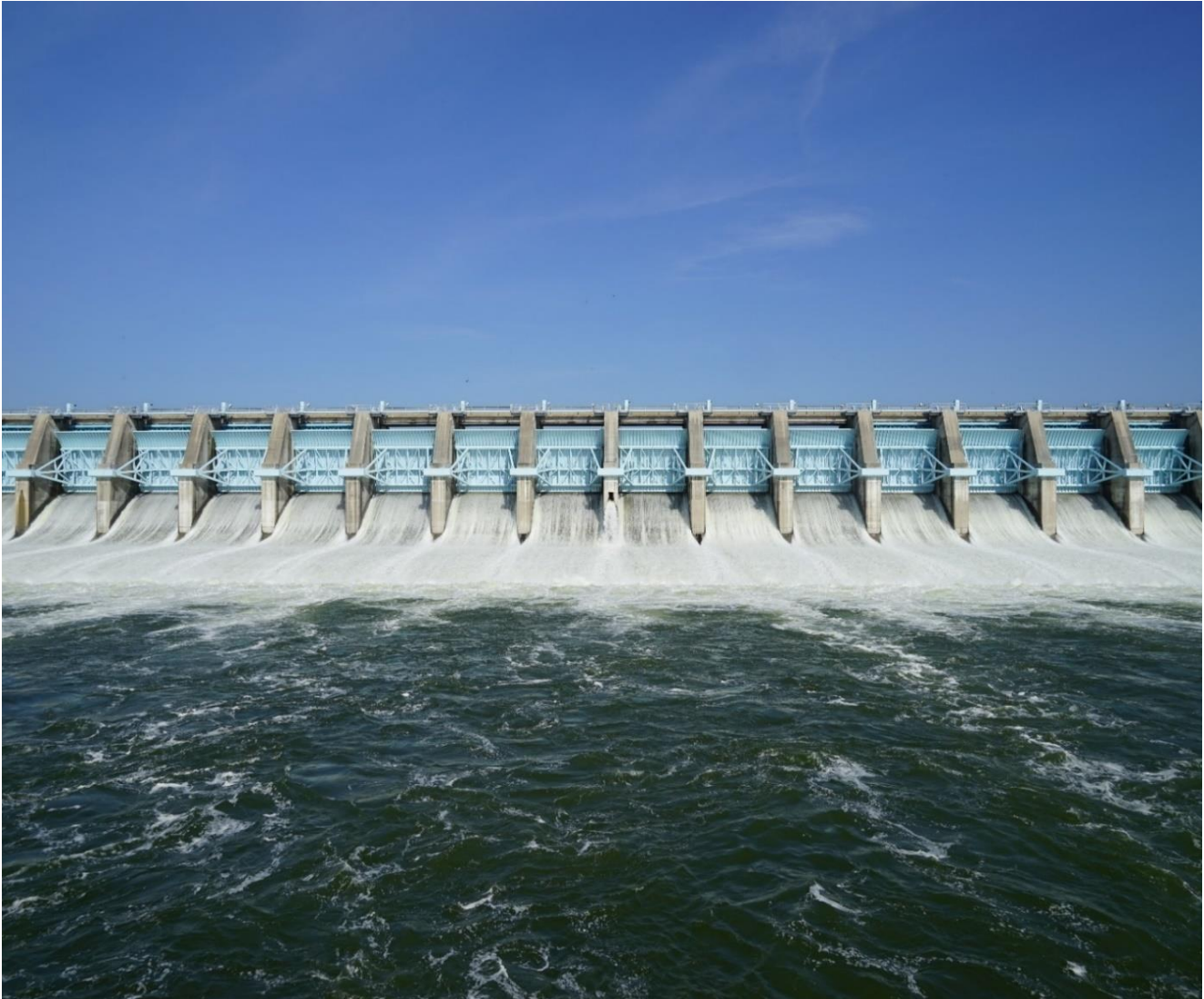
Spillway at Richland Chambers
