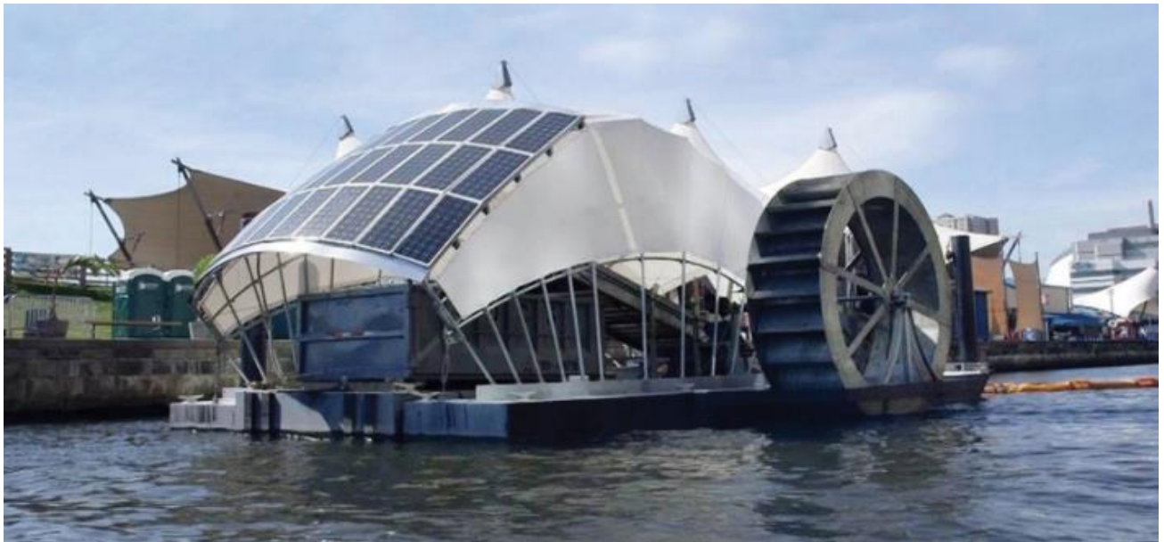
Pictured above is a water wheel structure designed to pull trash out of our waterways.
