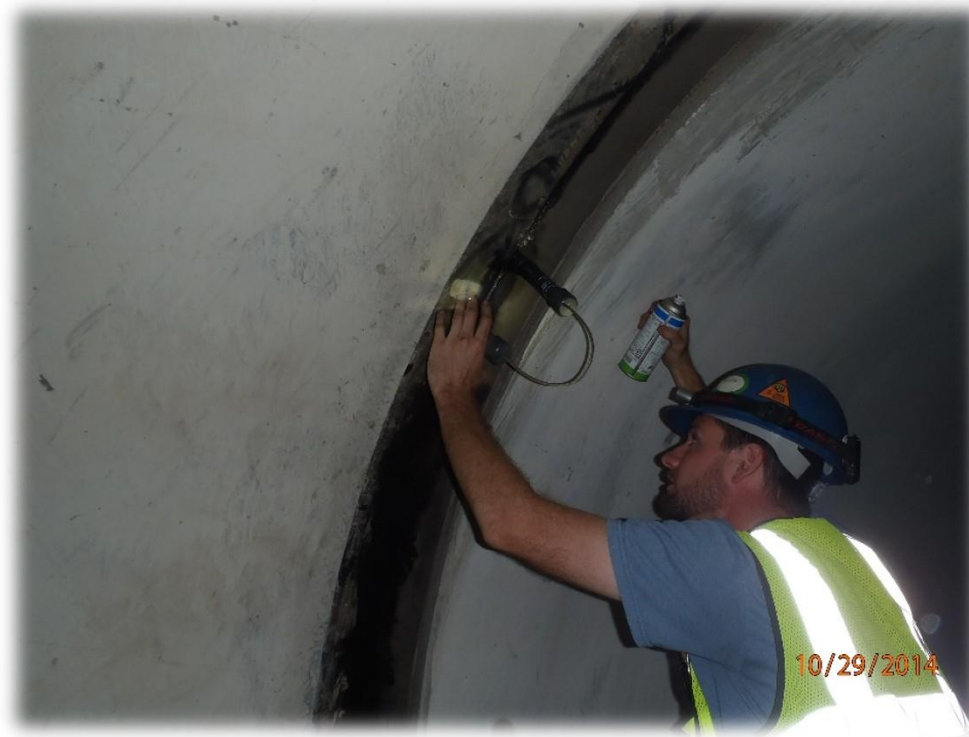
Certified Welding Inspection – Magnetic Particle Inspection steel Steel Inspectors
