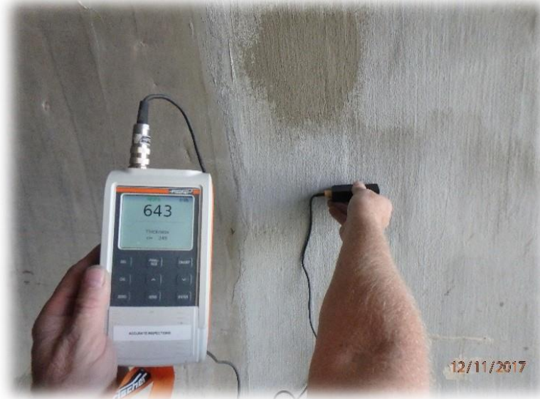
Pipe Quality Assurance – Cement Mortar Lining Thickness Verification Accurate
