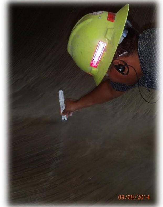
Pipe Quality Assurance – Cement Mortar Lining Thickness Verification Accurate
