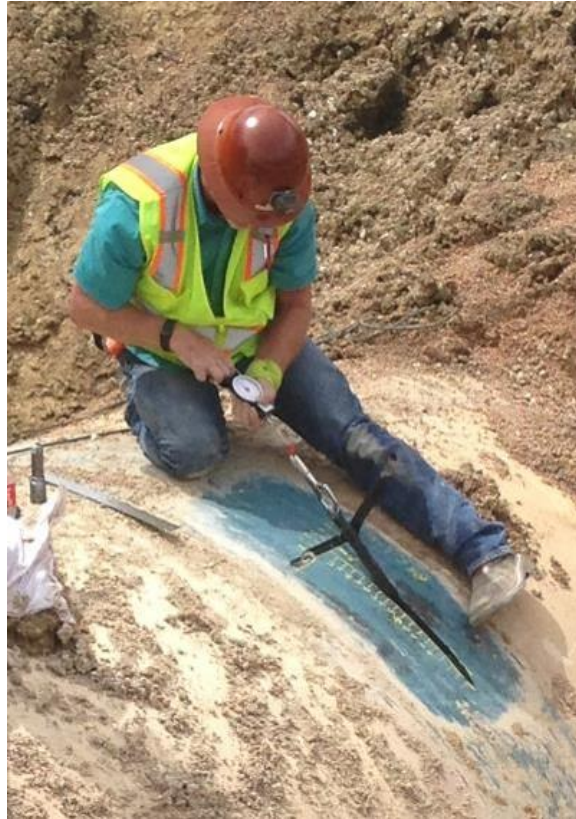
Coatings Quality Assurance – Weld After Backfill Joint Wrapper Proveout
