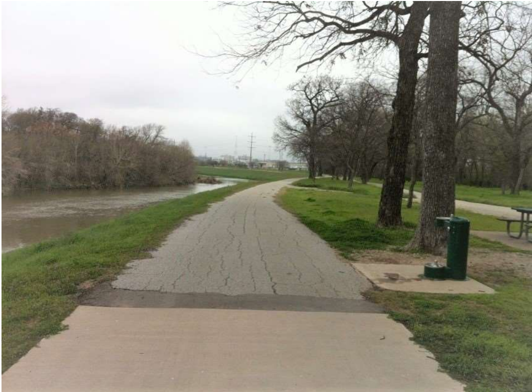
Trail resurfacing enhances the trails for safety and sustainability. Shown here is a resurfacing project that will replace the weathered asphalt.
