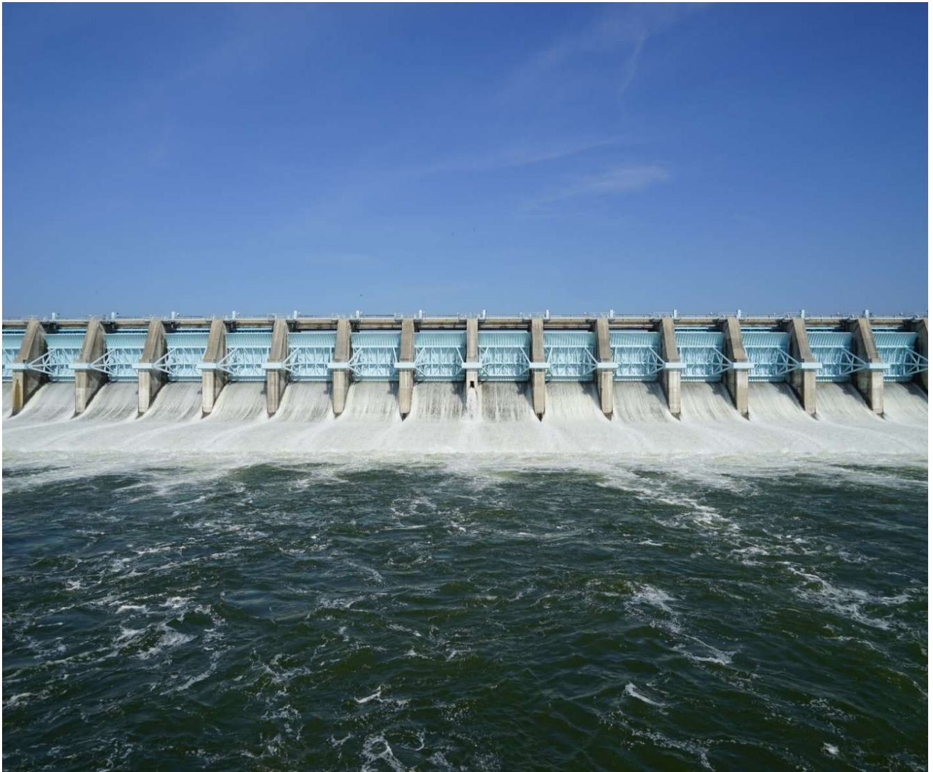
Spillway at Richland Chambers
