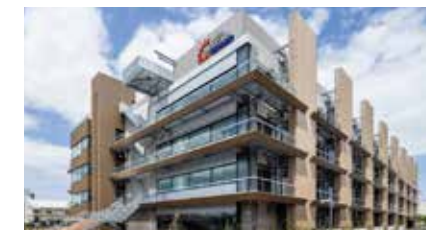
Mitsui Link-Lab新木場2
