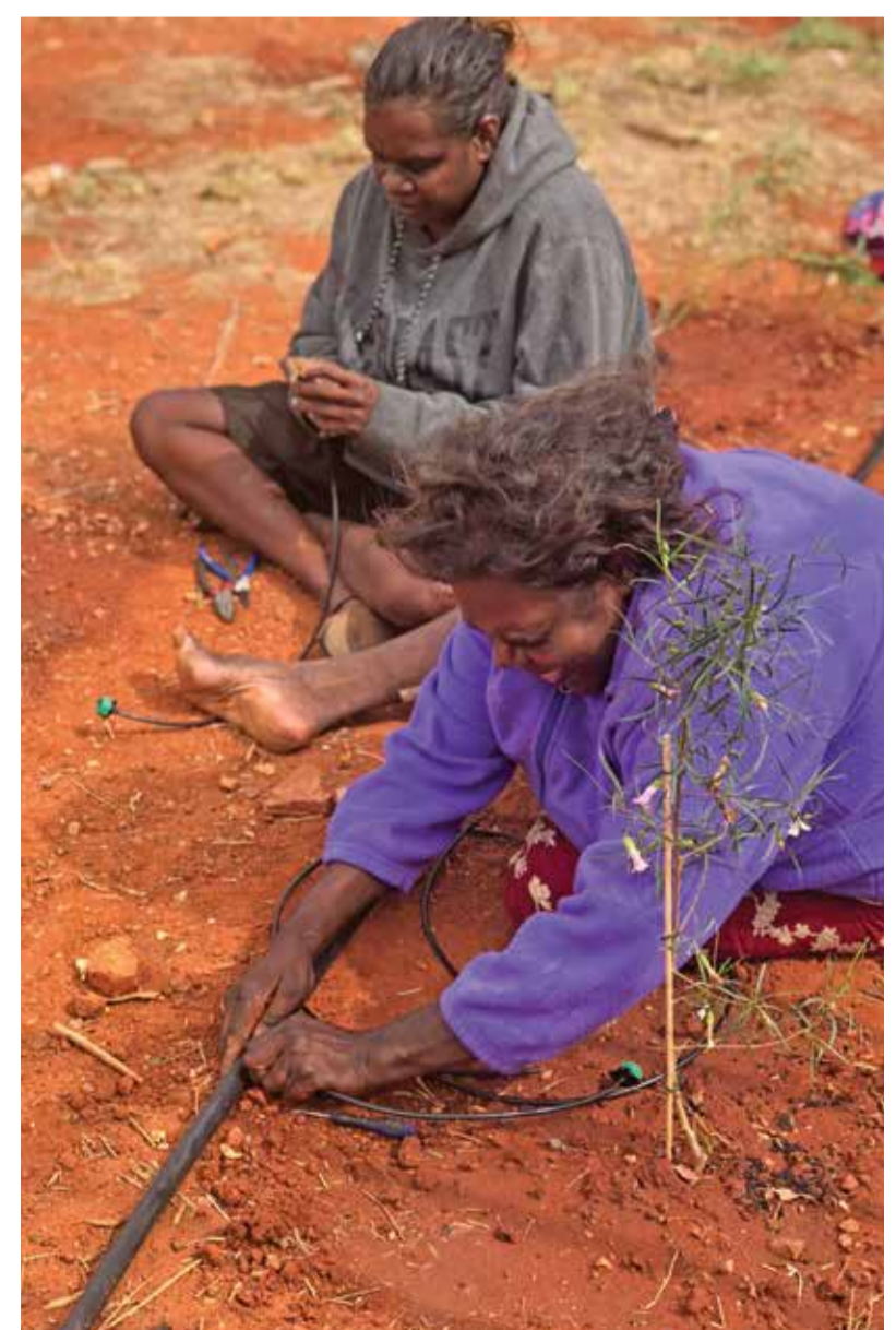
Magda Curtis and Latoya Curtis installed the reticulation.
