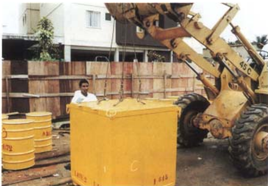
20. One of the specially made 5 tonne waste storage boxes.
