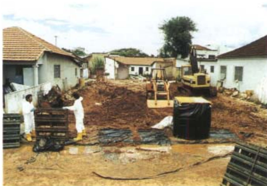
14. The same site after removal of the contaminated rubble.
