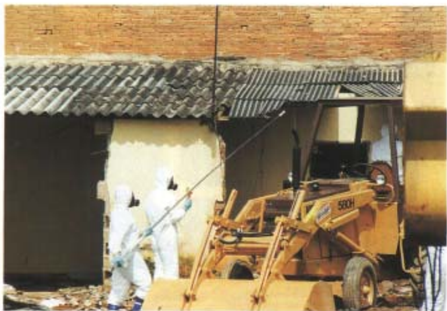
8. Monitoring the roof of the house of E.F.2 and S.F.1 during demolition.
