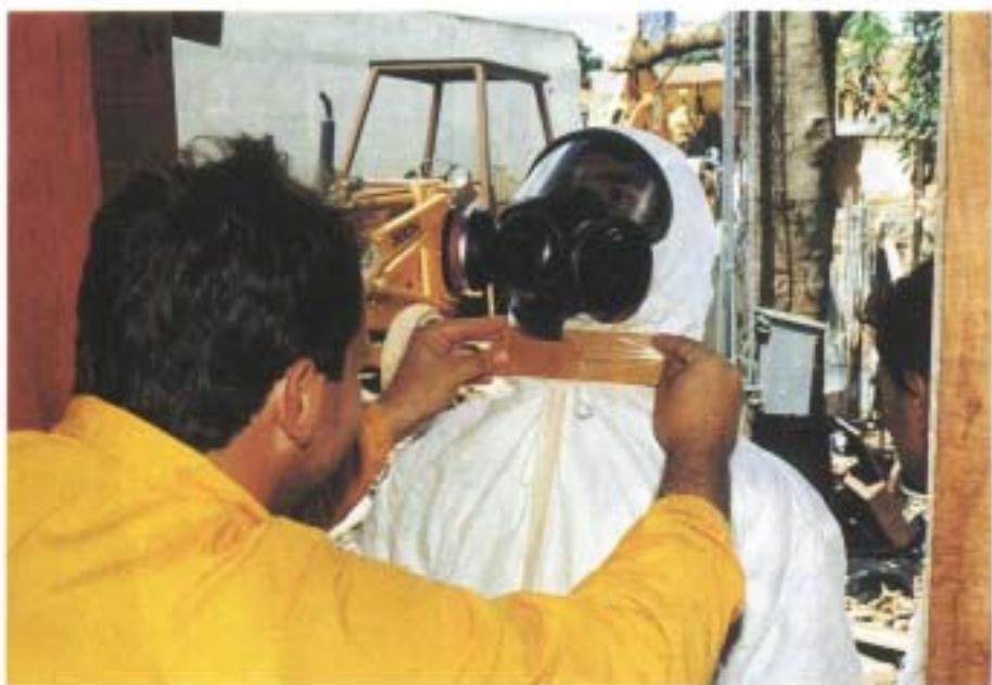
7. Preparing to demolish the house of E.F.2 and S.F.1, near Junkyard 1.
