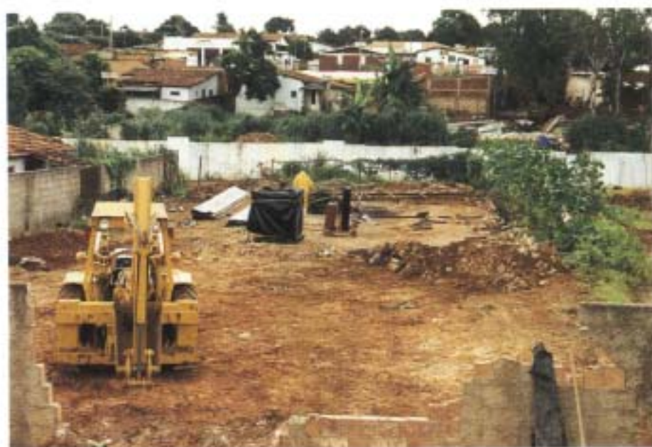
11. Clearing the site at Junkyard II on 6th Street.
