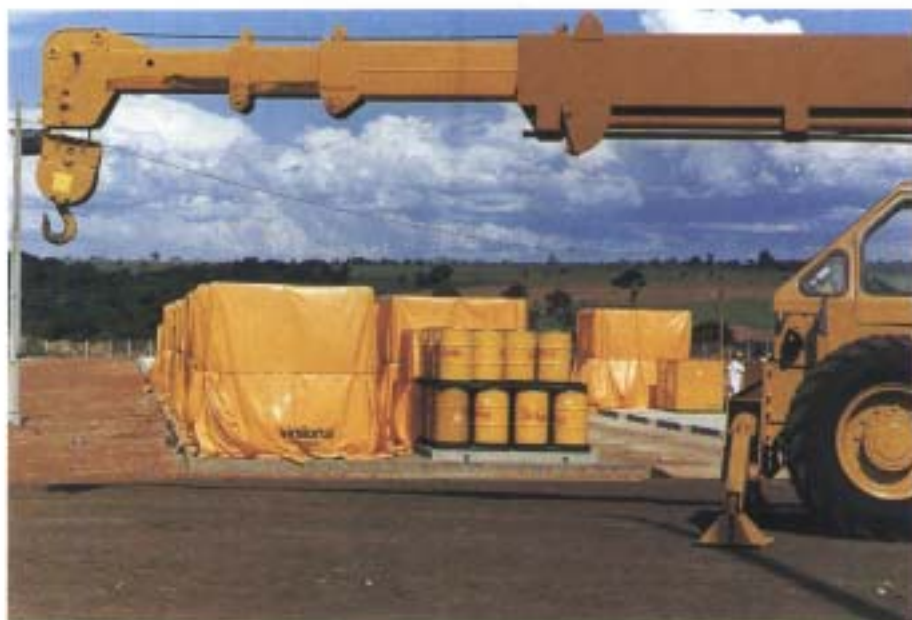
23. Boxes and drums of waste stacked and covered at the temporary storage site.
