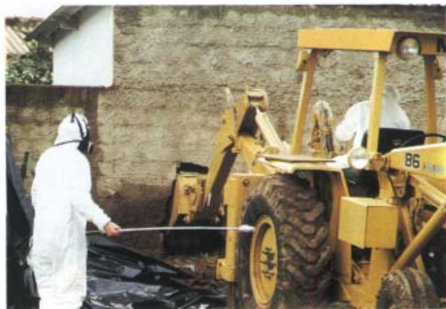
10. A hole is made to remove a radiation hot spot giving a dose rate of 0.5 \text{ Sv}\cdot\text{h}^{-1} .
