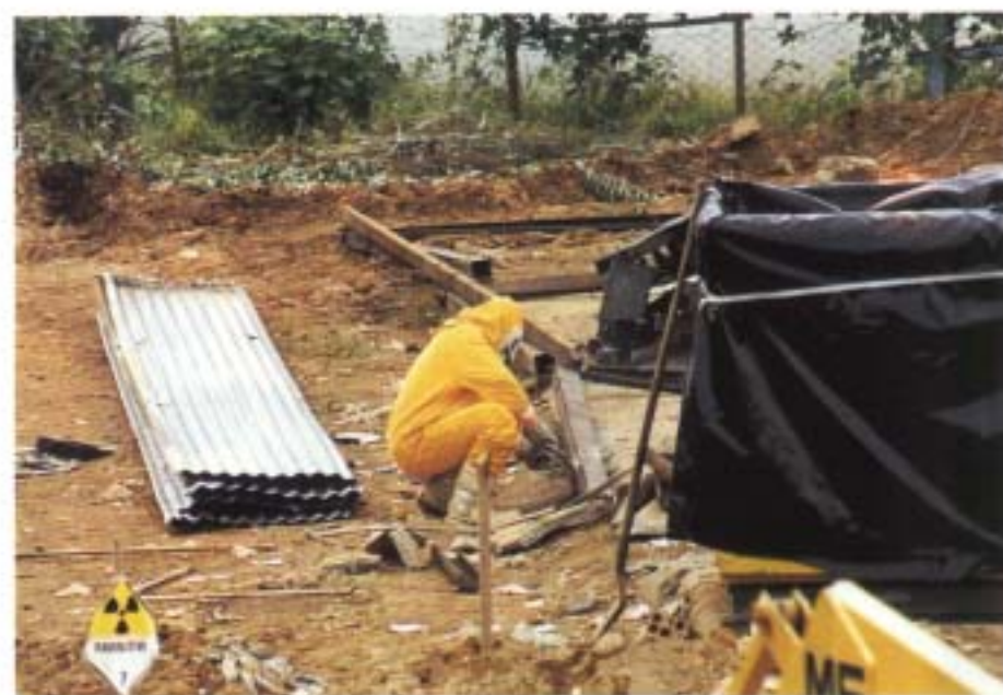
12. Junkyard II: cutting up contaminated girders.
