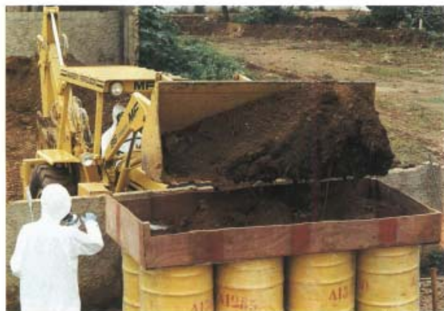
18. An improvised way of filling eight drams simultaneously with contaminated soil.
