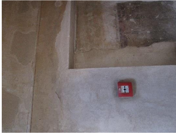
Figure 5. Fire alarm system in Ali Qapu Pavilion
