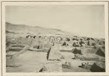
FIG. 273.—STOREHOUSES WITH BRICK VAULTS IN THE RAMESSEUM. ( Phot. Baraize. )
