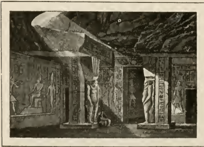
FIG. 411.—SANCTUARY OF THE TEMPLE OF TIRHAKAH AT NAPATA (After Cailliaud).
