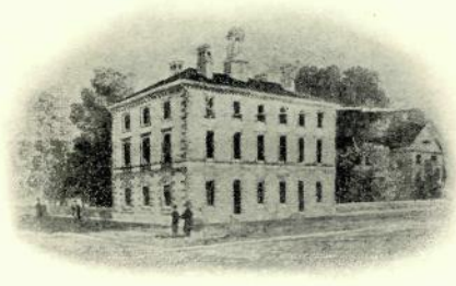
LAWRENCE INSTITUTE First building, erected 1848-49
