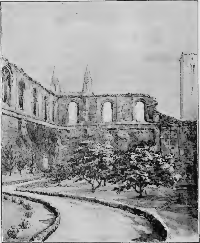
THE SOUTH WALL OF THE CATHEDRAL
