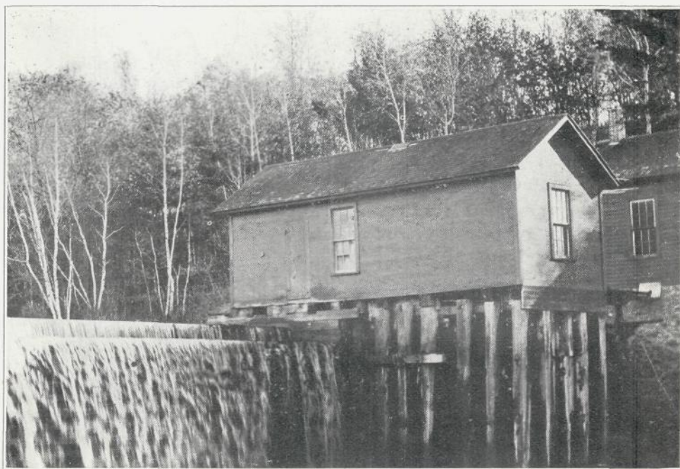
THE BURKHARDT MILLING AND ELECTRIC POWER PLANT
