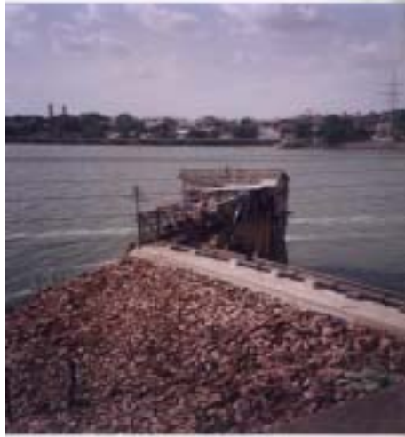
Plate.3.1 Pumping Station at Kamala Park (U.L)
